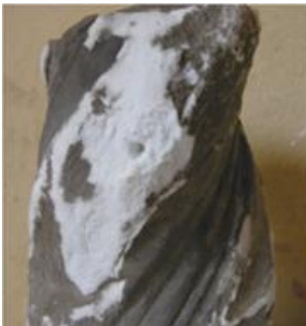
Heavy decayed fragment of a marble column
